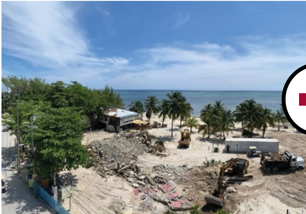
TEAR DOWN AND SITE PREP
